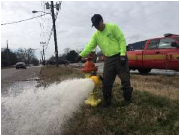
LFD Lt. Dusty Helton flushes a fire hydrant on Greenville St.
