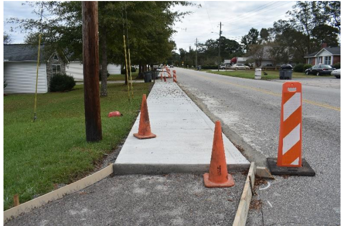
Sidewalk Construction at the Corner of Ragland and Colquitt Streets
