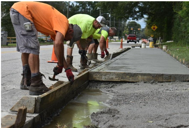
Crews Constructing a Sidewalk on Ragland Street
