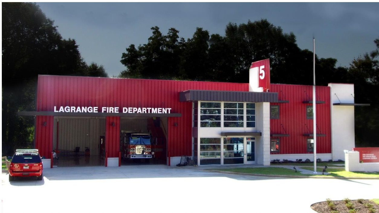
LaGrange Fire Station #5
