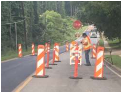
Crews continue to work on Country Club Road improvements
