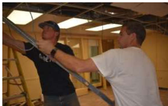
Crews worked over the weekend to make the changes
