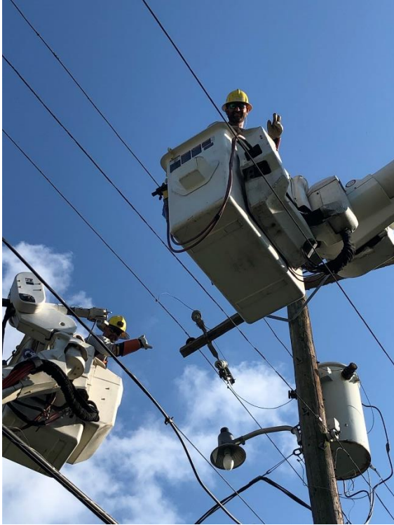
City of LaGrange Utility Workers in Louisiana
